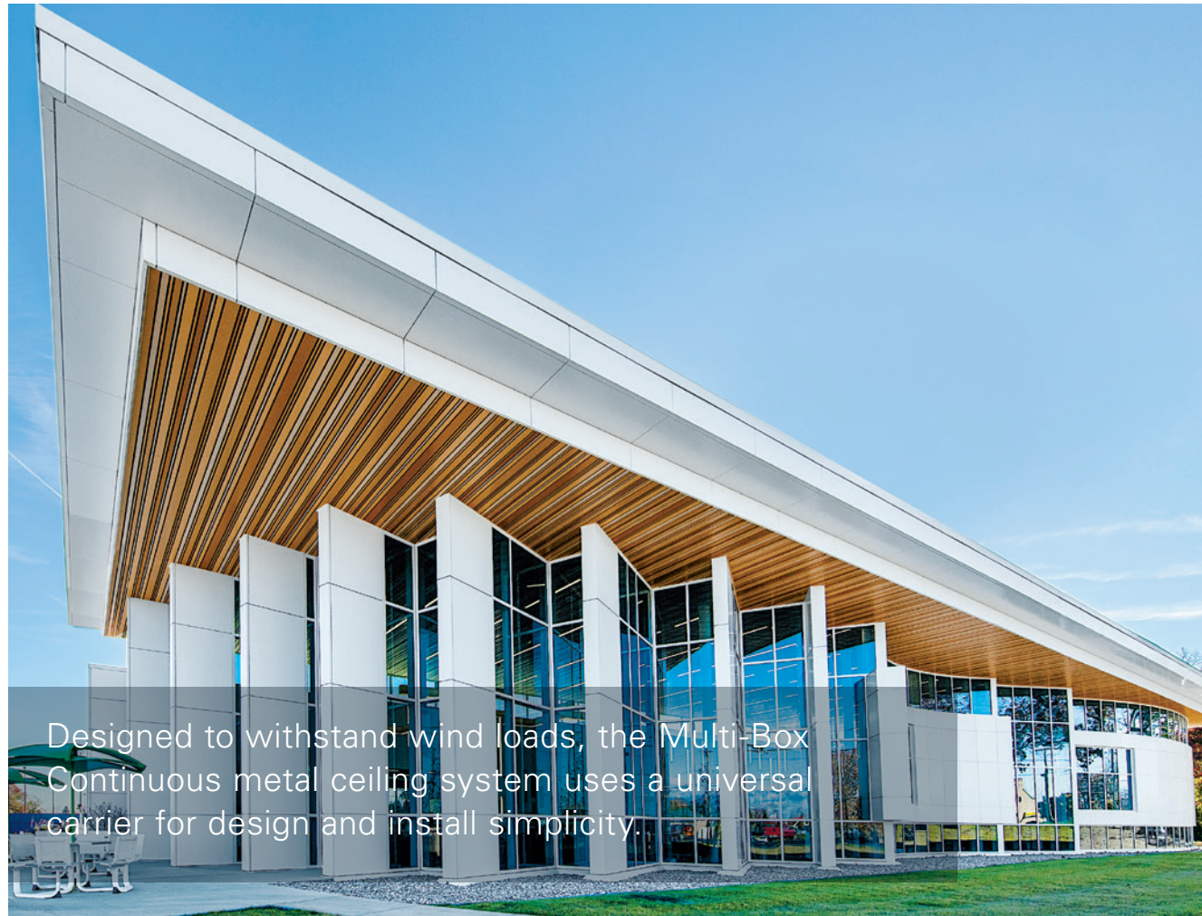
Project: King Road Branch Library, Toledo, OH; Multi-Box Continuous – Exterior Photo credit: Bob Perzel
