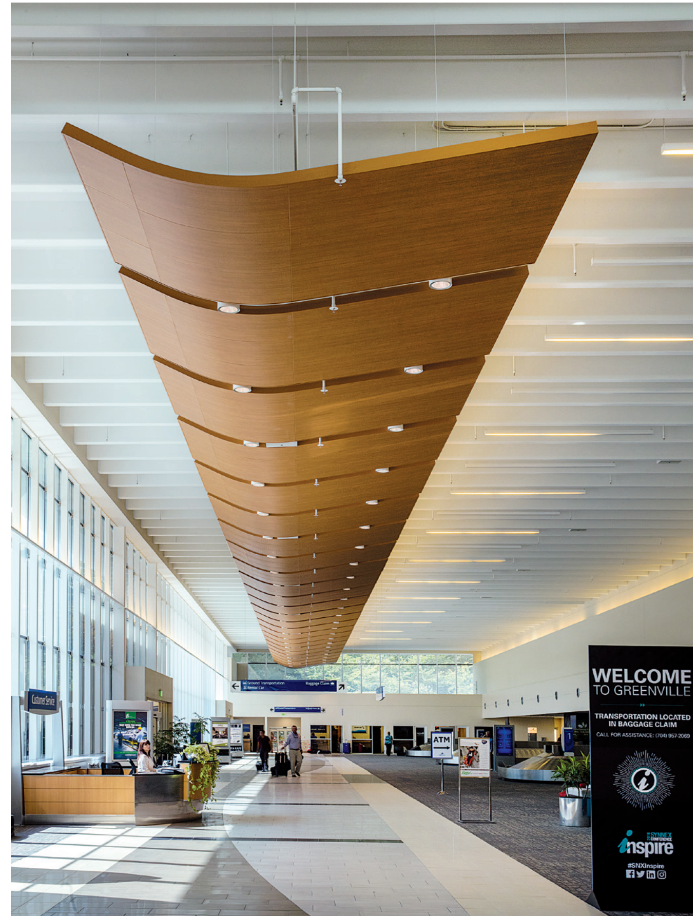
Project: Greenville-Spartanburg – GSP Airport; Torsion Spring – Curved Photo credit: Bob Perzel
