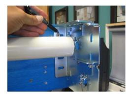
Place the end plug into the bracket and mark the location for proper installation of the end plug bracket.
