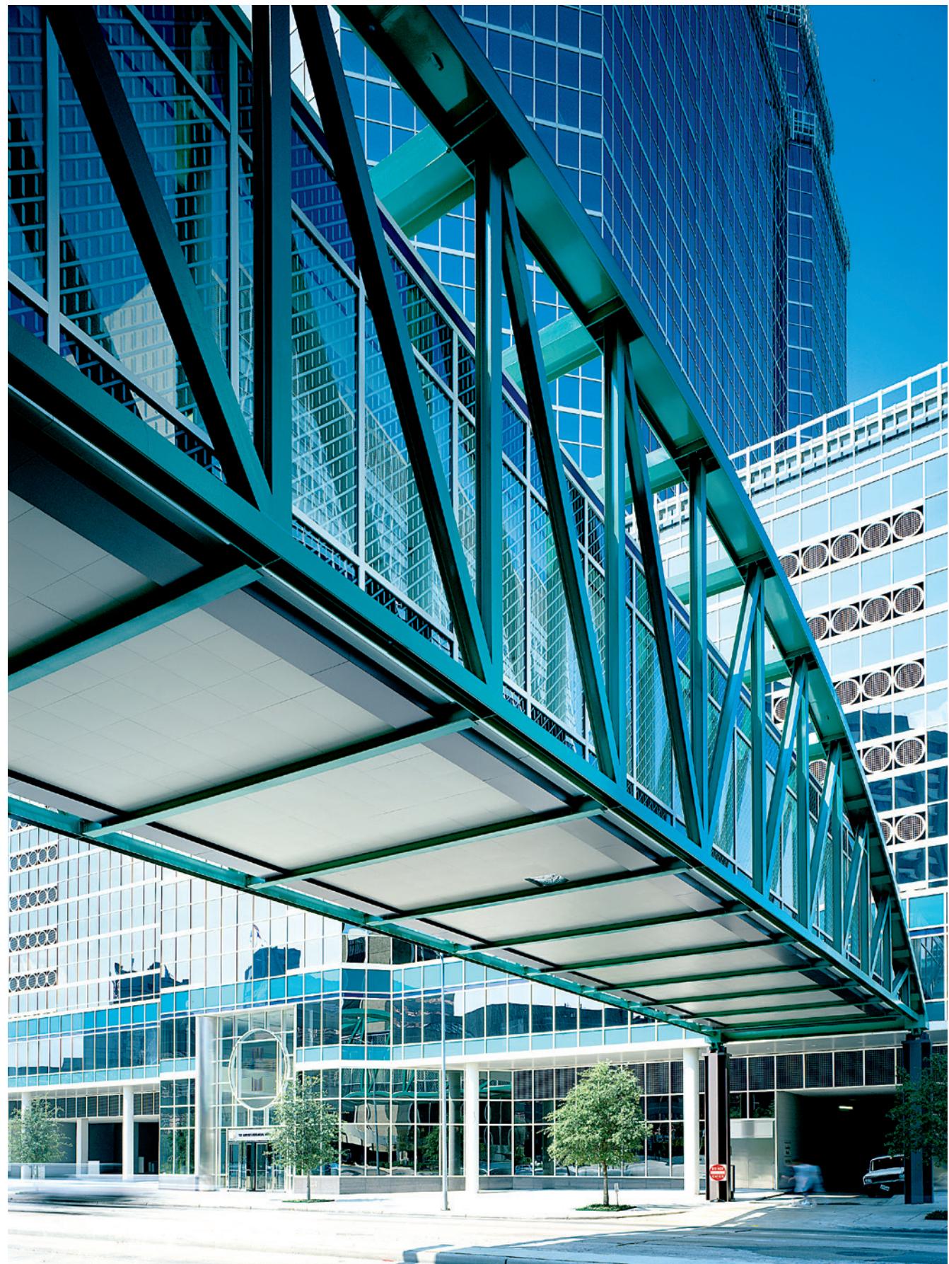
Project: St. Luke's Professional Building, Houston, TX; Exterior Plank
