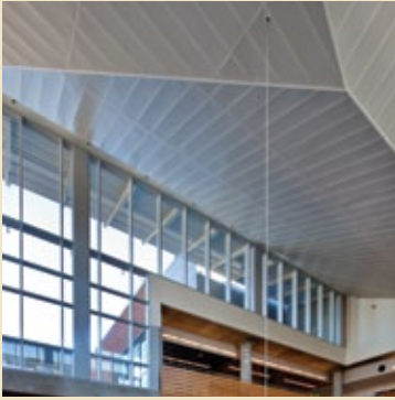
Above, Left to Right: Georgia Tech Clough Commons, Atlanta, GA Architect: Bohlin Cywinski Jackson Product: Hook-On Photo Credit: Bob Perzel
