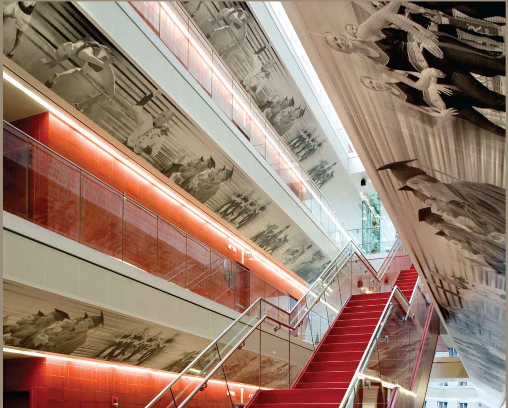
Front Cover: San Jose Airport, Terminal A Architect: Skidmore, Owings & Merrill LLP Product: Nysan Skylight Systems
